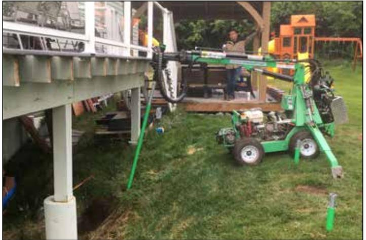
**Working next to the existing deck** - We can stay on the ground and reach over a low deck to install the piers through the existing framing.
