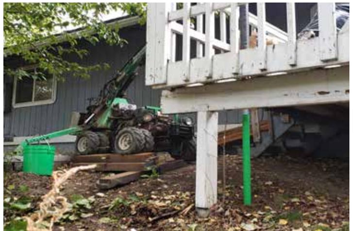
**Working from an existing deck** - Our R2D machine is only 1500#, so if the deck is stable enough we can work from the decking itself.
