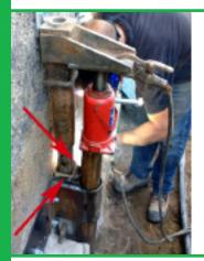
**Step 10:** Install the jack support system and put the system under pressure. Subsequently, weld the footing bracket on each side of the wall bracket (see arrows for the location of welds).
