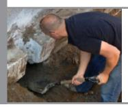
**Step 3:** Clear 8" of ground below the footing. Ensure the bottom of the footing is flat and smooth to allow full contact with the bracket.
