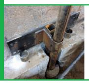
**Step 6:** Place the pier in front of the footing bracket and insert the wall bracket in the footing bracket coupling and in the Techno Metal Post. Be sure to maintain a mimum distance of 3-4" by placing the wall bracket on two couplings and against the wall.
