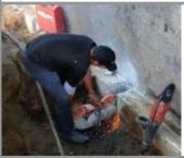
Step 2: Cut a 6" section out of the existing concrete footing (this may be wider if using a different bracket). Chip/clean the face of the stem wall to create an even plane on the stem wall to bottom of footing.
