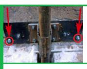
**Step 7:** Using two concrete anchors, 3/4" x 8" long, set the wall bracket on the concrete foundation wall, making sure to install it level.
