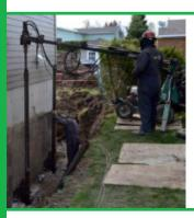
**Step 8:** Install the Techno Metal Post in the ground until refusal or until torque values required by an engineer are reached.
