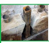
**Step 4:** Insert the footing bracket under the foundation wall;
